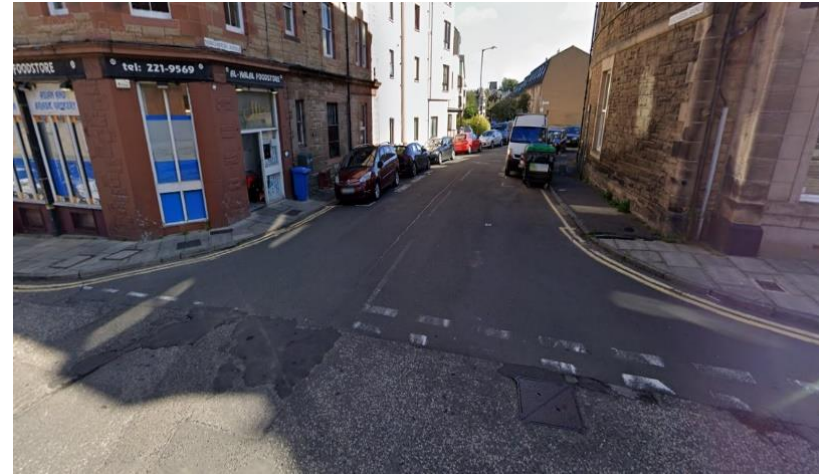
Photo of the junction after the width has been reduced and tactiles and dropped kerbs have been installed
